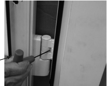
This will release the hinge cover.
